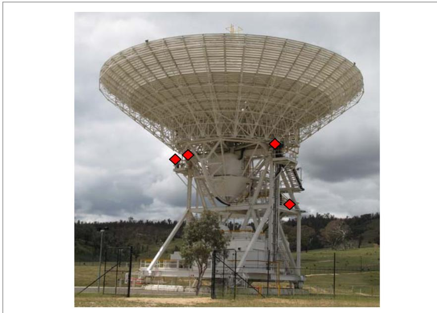
*Figure 6: VLBI Azimuth rotation - survey target positions on telescope structure*
