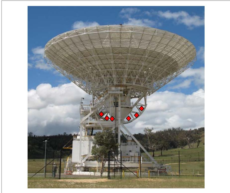
*Figure 8: Elevation rotation - survey target positions on telescope structure*
