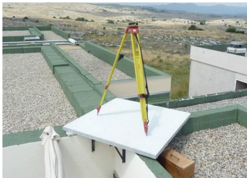
Concrete pad on the roof
